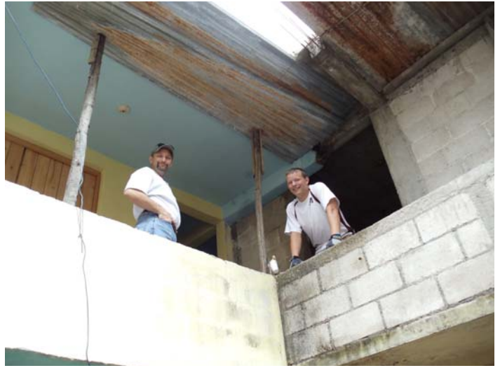
Toby and Peyton ready to build doors in San Pedro.
